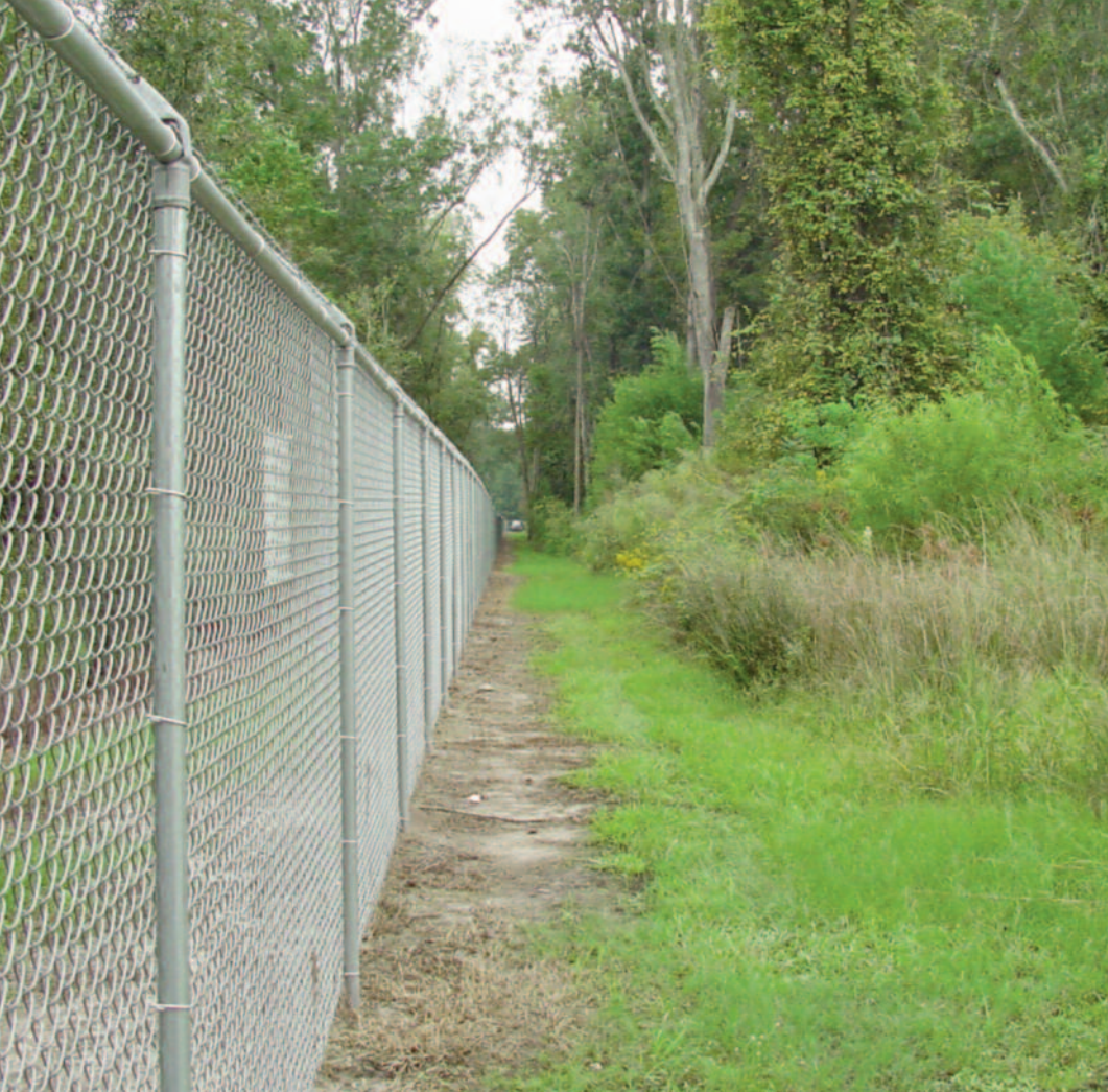
Left: Perimeter fence at Savannah Air National Guard Base, Georgia. Some natural resources projects can be justified also on the basis of security needs. For example, clearing of undesirable vegetation along the base perimeter is often funded using security funds, rather than environmental ones, because of the importance of maintaining an open roadway along perimeter fences for security purposes. (Photo: Douglas Ripley)
